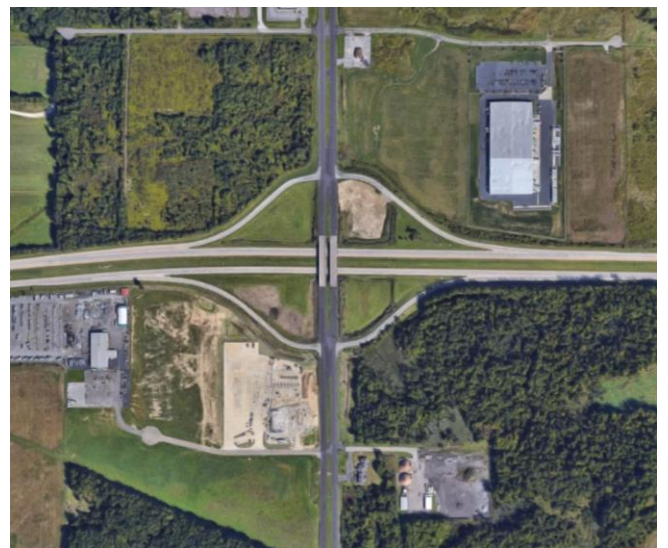
Figure 8: 2018 Aerial of Bailey Road / IR 76
