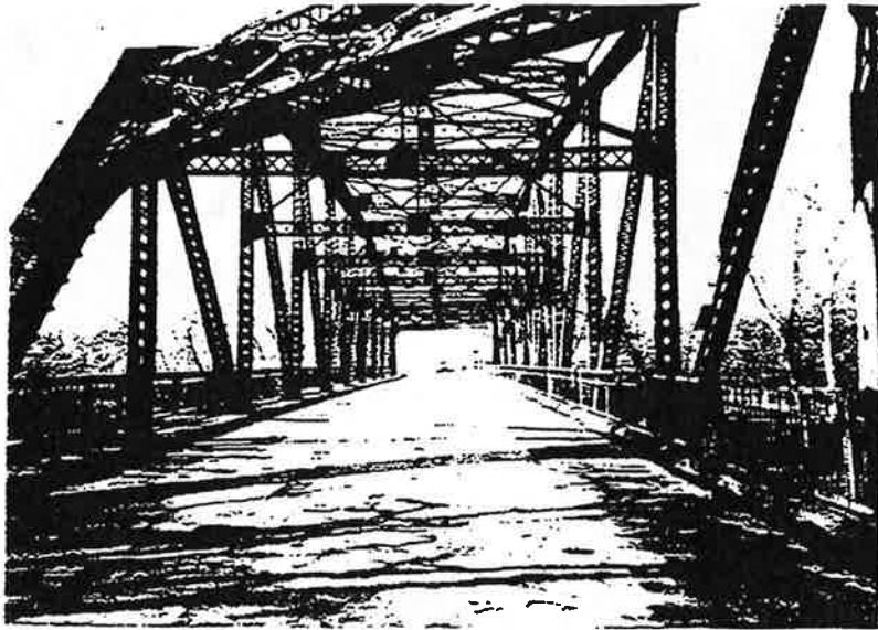
TYPICAL TRUSS SUPERSTRUCTURE VIEW
