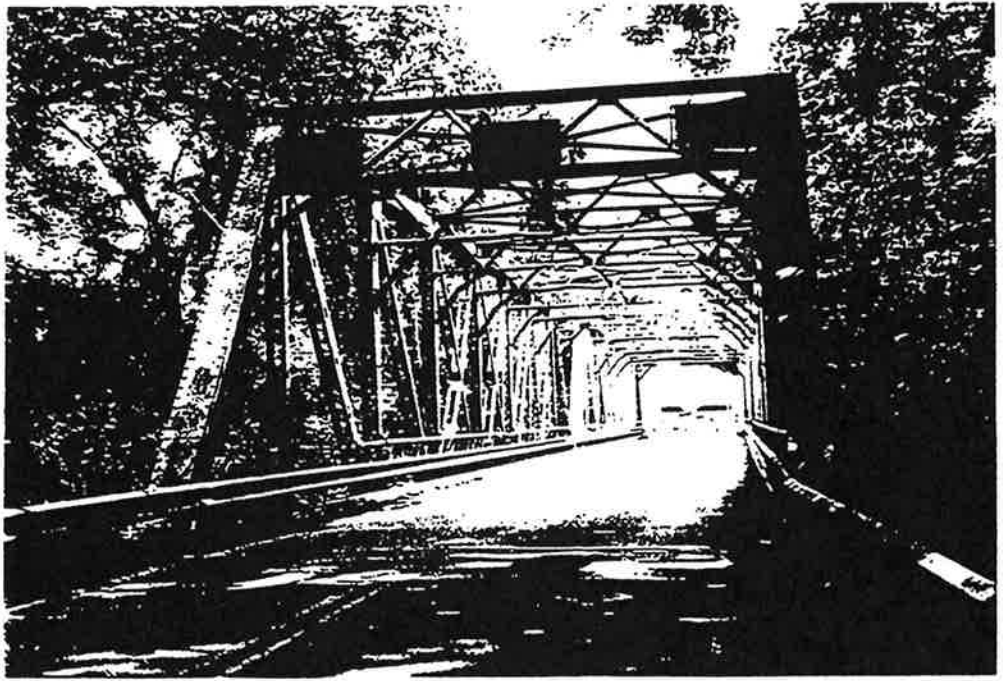
Photograph 2: Mt. Jackson Road Bridge. View Facing West.
