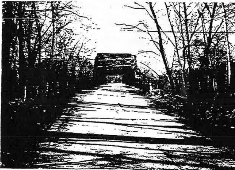
FAR APPROACH ROADWAY
